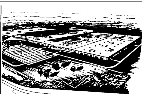
NISSAN MANUFACTURING FACILITY in Smyrna, Tennessee
